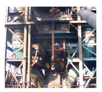
The Hydraulic Distributor design includes a reliable and effective shower water cooling system with a proven operating record of reliability under extreme blast furnace top conditions.
